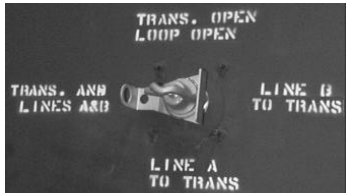
Figure 26. V-blade switch.
