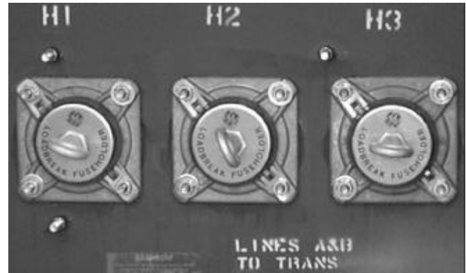
Figure 9. Loadbreak fuses.
