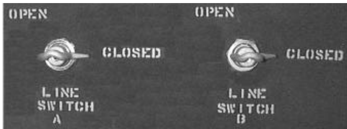
Figure 18. Loop-feed switches.
